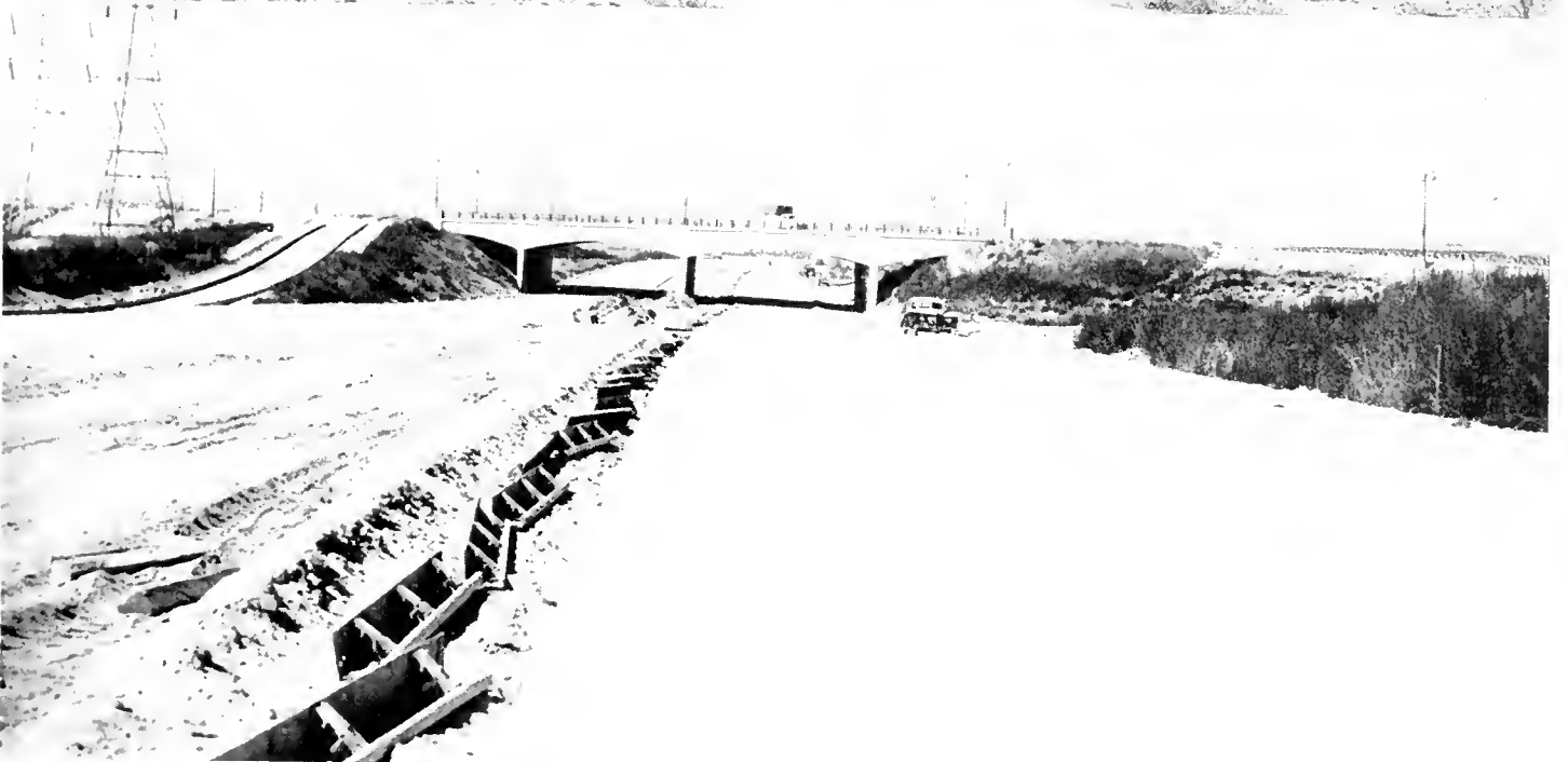
UPPER: Looking northerly toward Atlantic Avenue Undercrossing. The pavement on main traffic lanes of freeway has been completed, and construction operations are in progress on the side collector roads and ramps. CENTER: Looking easterly along Dominguez Street showing, on left, steel girders in place for Pacific Electric grade separation and on right steel girders in place for Union Pacific Railroad grade separation. LOWER: Looking southerly along Long Beach Freeway showing the overpass bridge carrying Long Beach Boulevard over the freeway. Northbound on-ramp from Long Beach Boulevard shown on left.
